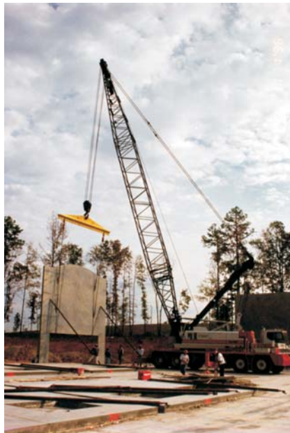
International Airport Center
